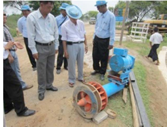
Hydropower Turbine being installed near Mandalay
