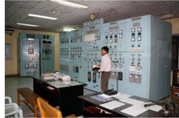
MOEP Substation Installation near Pathein
